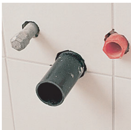
3. Start to knock out (with the point of the tile hammer) the hole in the middle and continue outwards. That way you can easily enlarge the hole diameter.
